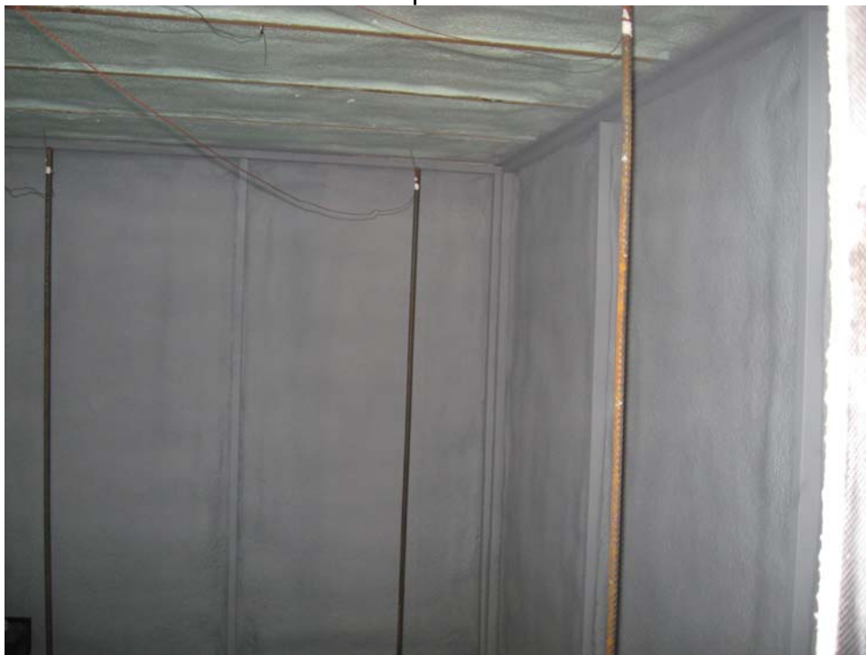
Photo of ceiling
